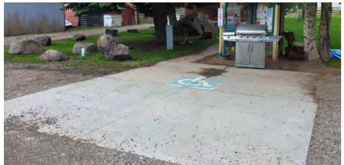
Ex. Accessible Parking Space at Town Park
